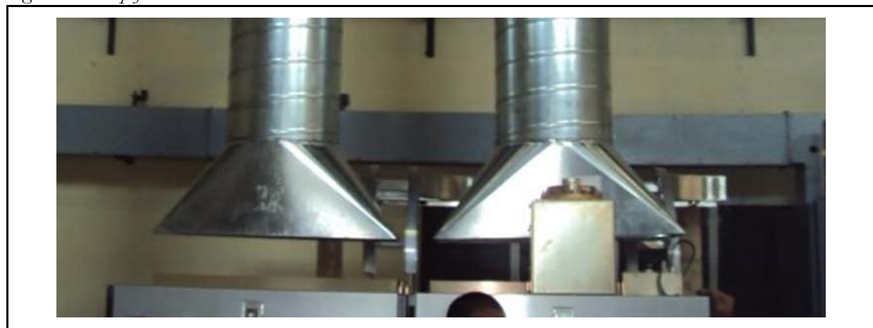
Figure 4.3: Gap for Exhaust Air
